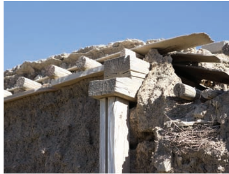
Beam, column detail of the Maitreya temple
