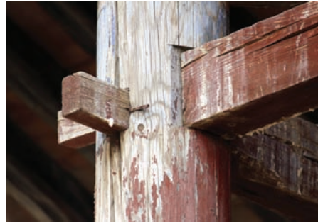
Half-sill joining at the external column and beam hanging at a girth
