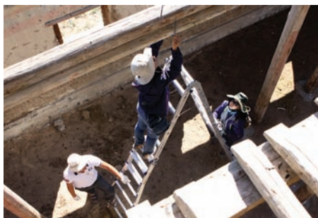
Measuring the lower cross beam and members connecting columns
