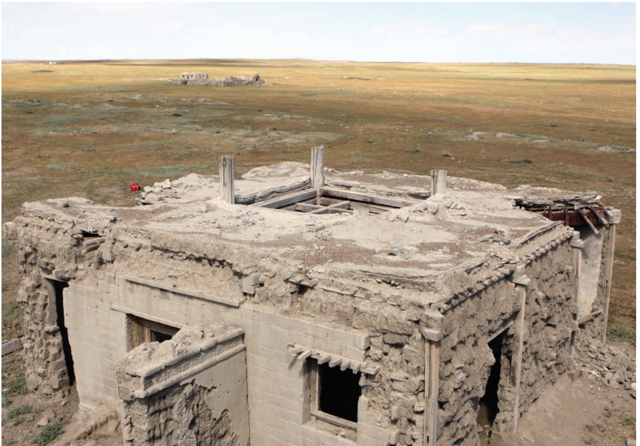
Roof status of the Maitreya temple
