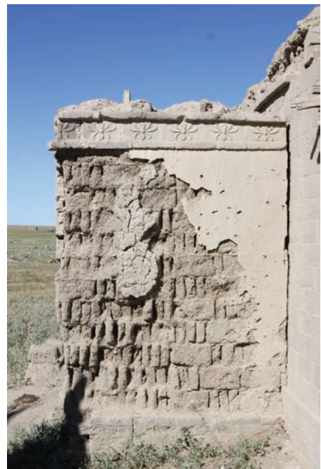
Wall on the right of the front room
