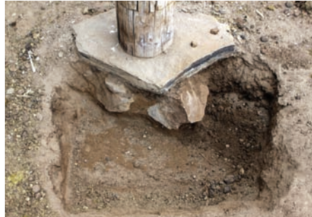
X5Y2 corner stone trench inspection
