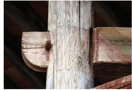
Dado-joint at the external column and beam hanging 45 degrees at a corner
