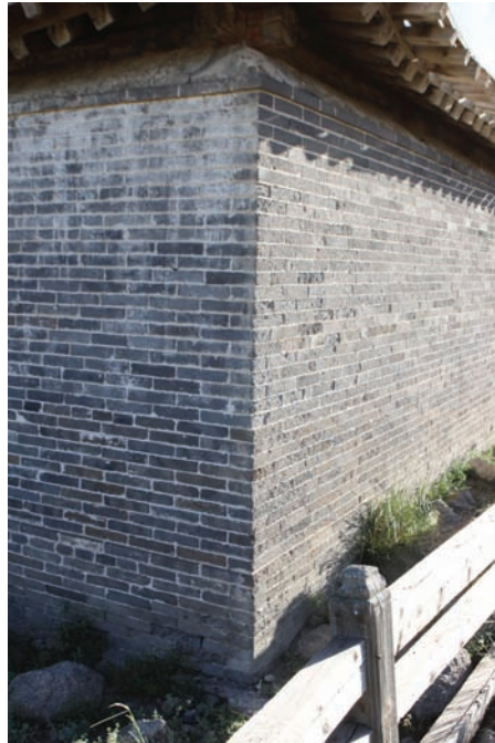
Exterior of the wall
