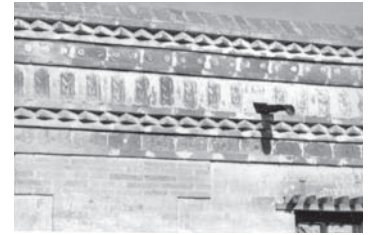
Roof handrail of the Maitreya temple (1981)
