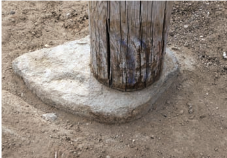
Exposed natural foundation
