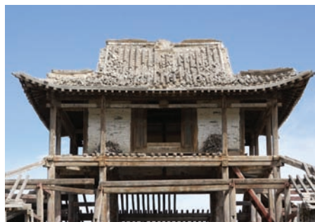
Entrance in the middle of upper story as viewed from the outside
