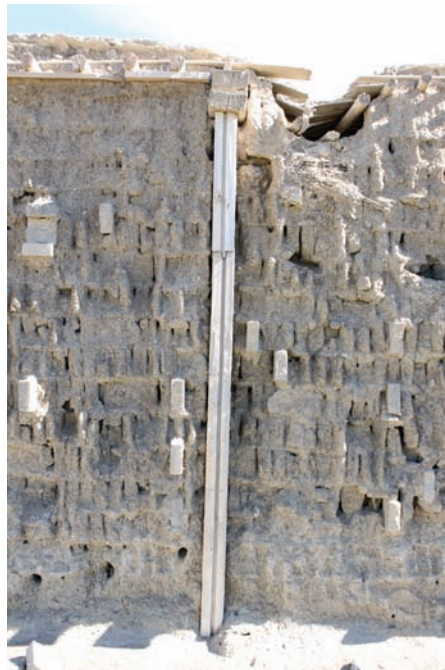
Exposed wall interior column
